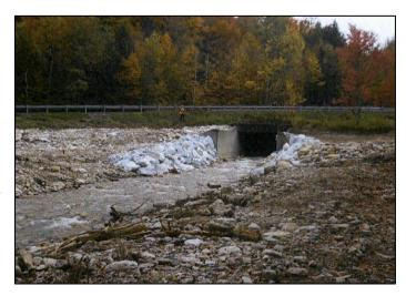
**Figure 3.1:** Repairs to washed out wingwall abutment and retaining wall at the outlet of a Route 7 culvert near the Glastenbury-Shaftsbury town line.
